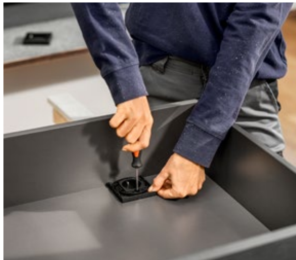
② Secure the outlet in place to prevent it rotating.
